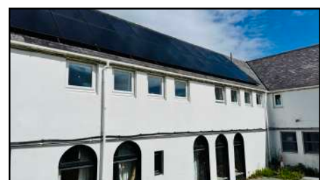
Above: Solar panel installation complete.
