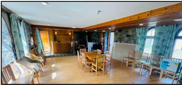
The rear dining room - still a work in progress - a bar has been constructed at the far end.
